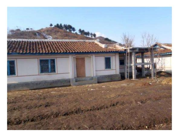
At Mopung, thermal isolation for houses will be provided, as well as solar water heaters. The concrete support for the SWH was in place, the systems are not yet delivered. Please note that low-temperature concrete is not easily obtained in DPRK; by consequence, activities are suspended in winter time. Also here, the SWH support structure dims the light at the nearby window.
